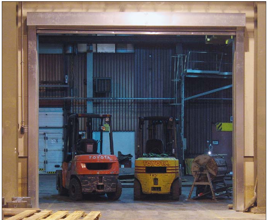
Large-sized doors allowing the passage of lifting machines. Miilukangas Oy, Raahе
