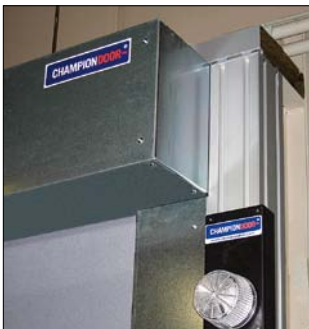
The upper housing of a roll-down fire door
